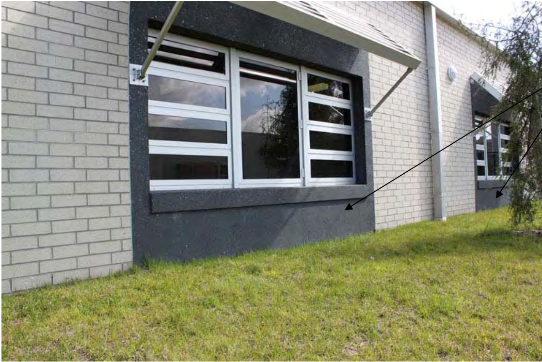
Close up of one window surround with Granyte
