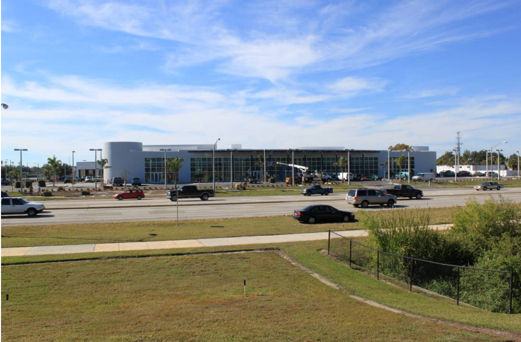
Dealership nearing completion (all pictures are prior to completion)
