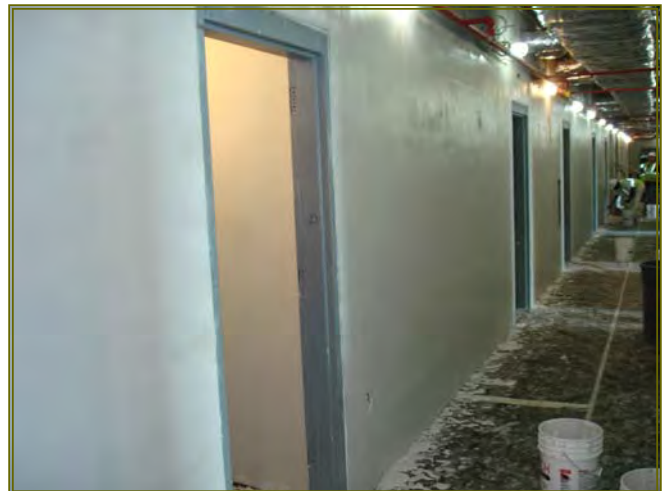
CMU construction after SKIMM application
