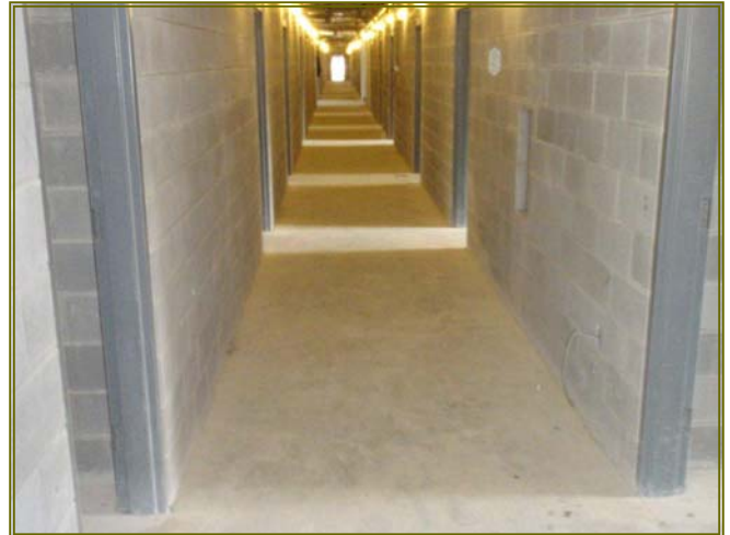
CMU construction awaiting SKIMM application
