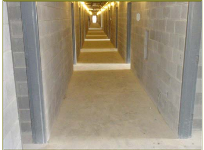
CMU construction awaiting SKIMM application
