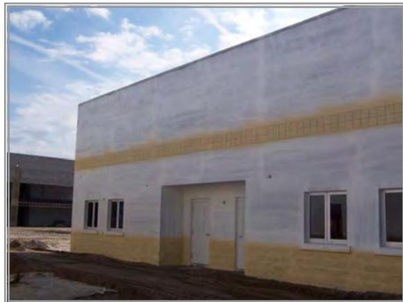
Contemporary CMU construction using REFORMIT as parging material. Buildings will be finished with Duroplex EXT.
