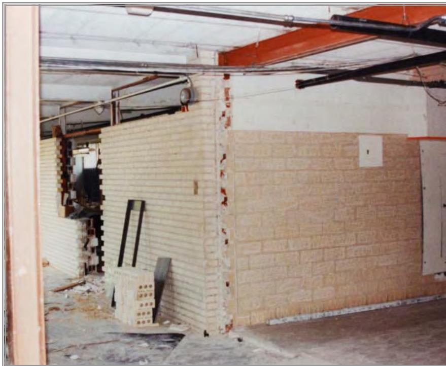
After a quick scarifying of only the glazed block, both the brick and block in this elementary school renovation will receive SKIMM™ to level and smooth the walls. The Duroplex® system will be applied as a finish coat.
