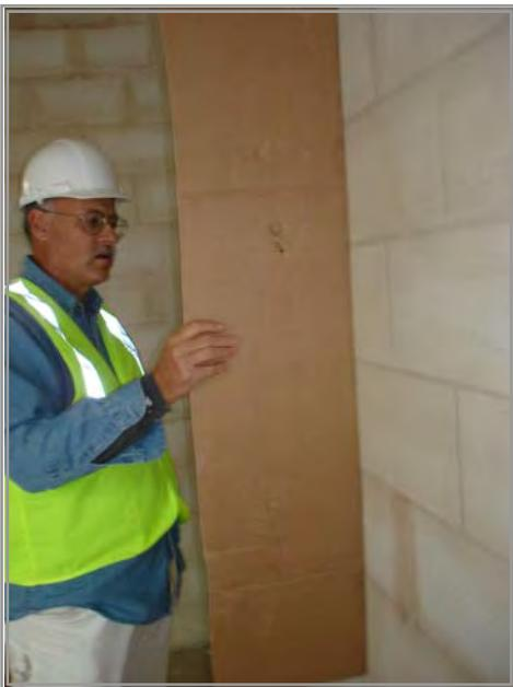
Moisture is still present in the SKIMM making the grout lines obviously still visible, but the CMU wall is smooth and flush to the touch. When the moisture evaporates in a day or two the grout lines will disappear. Plexture will be applied on top of the SKIMM
