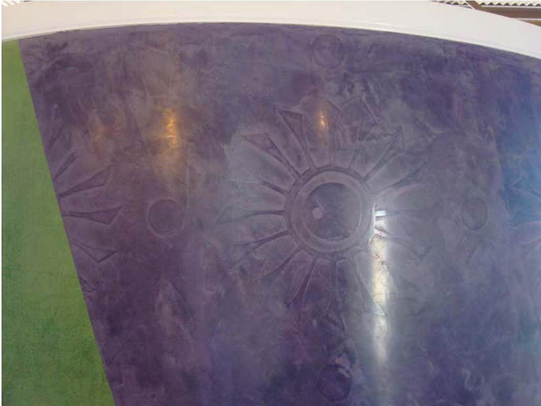
Spatula Stuhhi Venetian Plaster with embedded graphic
